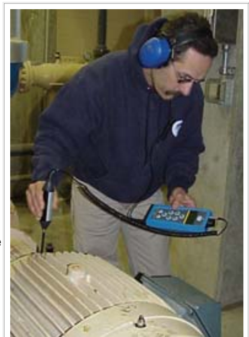
Dan Parry uses ultrasonic equipment to listen to pump bearings.
