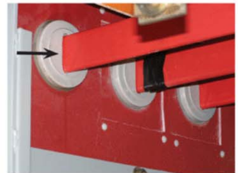
Figure 9b: Ultrasound was used to find corona on ceramic collars surrounding 13kV bus, no visible signs of corona are present.
