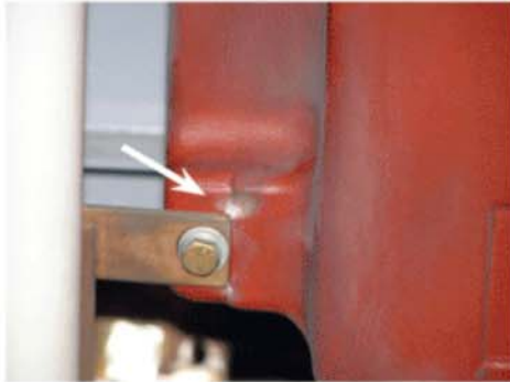
Figure 2 - A sharp edge on a piece of copper bus provides an excellent spot for corona activity.
